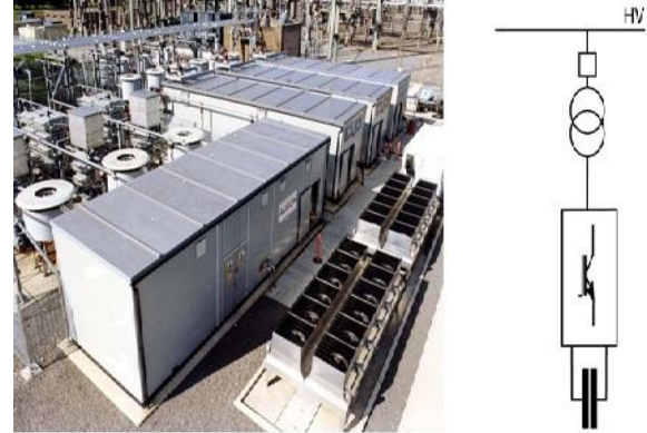
Fig. 3-Static synchronous compensator
